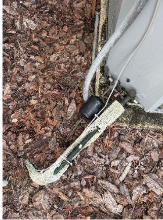
Torn Insulation of Refrigeration Line
